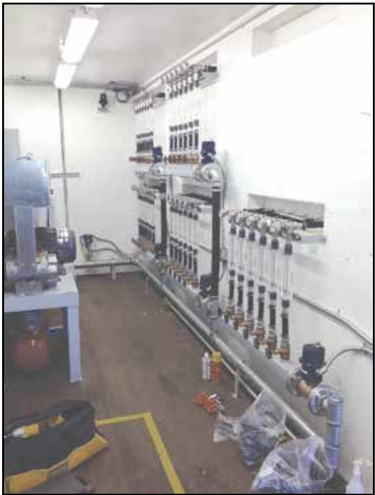
Air sparging system at Coos Head (photo taken from inside the trailer) Hoses run outside from trailer lines to the groundwater wells.
