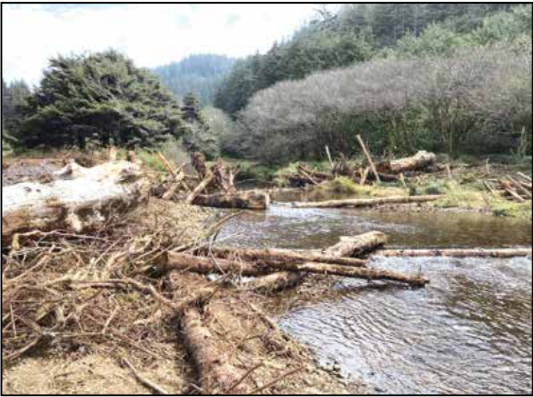
Ten “large wood” habitat structures were placed Big Creek. Large woody debris plays a vital role in stream systems, increasing stream complexity, providing cover for fish, sorting out spawning gravels, and maintaining floodplain connection at high flows.
