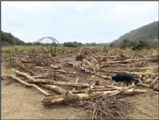
After floodplain excavation, large quantities of large and coarse woody debris were installed in the floodplain area. When flood waters spill into these areas, this material will slow the water and create complex, off-channel fish and wildlife habitat.
