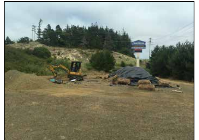
Jeremy Petrie operates the excavator to remove lead contaminated soils in an area identified from previous boring and test pits. Photographed by Janet Niessner.
