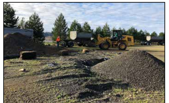
Jeremy Petrie loads tons of contaminated soil from a stockpile into trucks that will be hauled to a regulated landfill near Eugene. Certified clean gravel fills the excavated area. Photographed by Janet Niessner.
